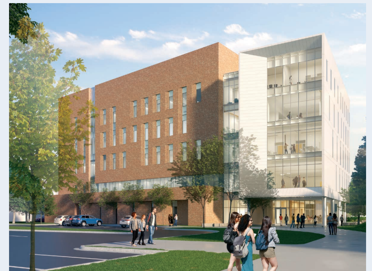
Rendering of the new UConn School of Nursing, opening fall 2026. (Digital rendering by Ayers Saint Gross)
